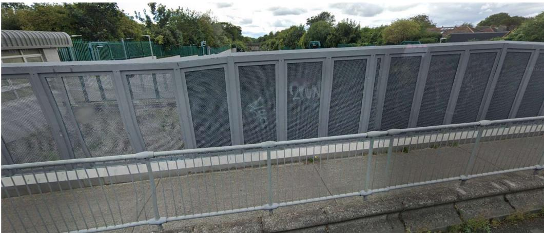
**Figure 4-8: Steel panels added to outer face of existing mesh screens (Middle Third Bridge, Killester)**
