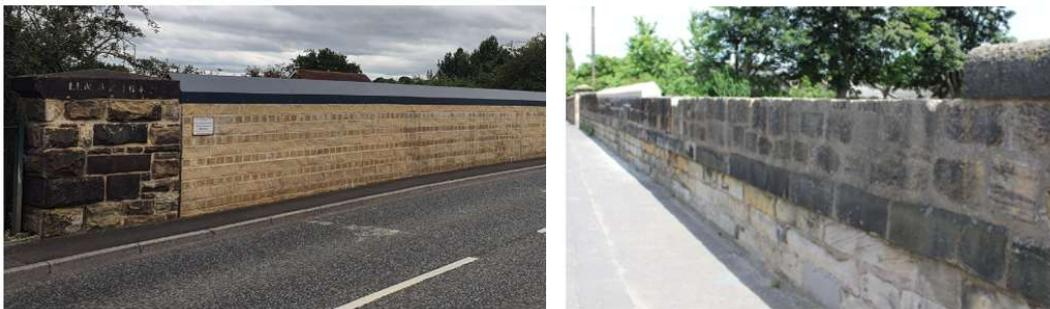
**Figure 4-3: Coping extension (GFRP coping – Stockton on Tees Junction (source:www.evergrip.com) and precast concrete – Borders Railway Project, Bonnyrigg Road Bridge)**
