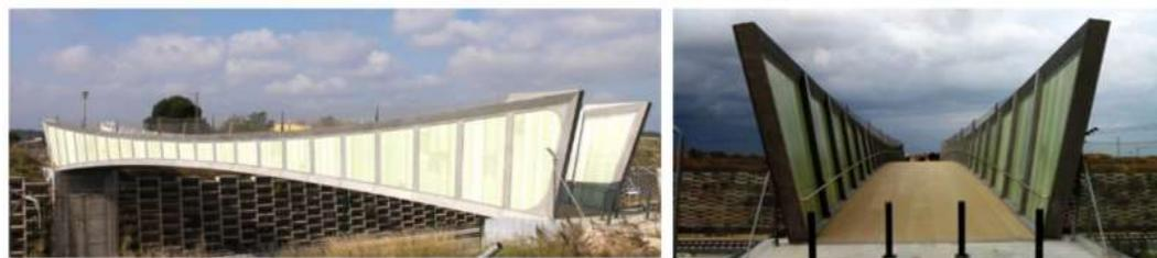
Figure 4-11: GFRP panels between chords of Vierendeel truss (Vilafant footbridge, Spain)
