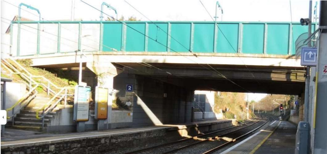
**Figure 4-7: Mesh infill replaced with solid steel panels (Raheny Station footbridge)**
