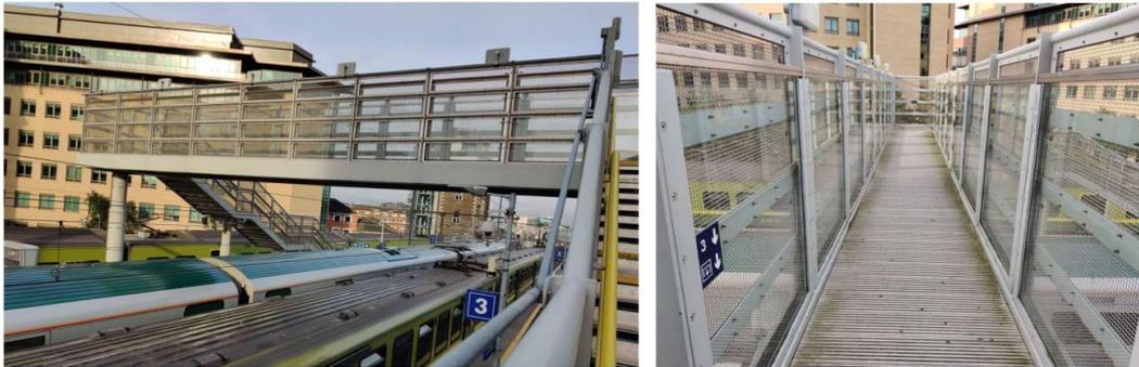
Figure 4-10: Clear panels on pedestrian bridge (Grand Canal Dock Station)
