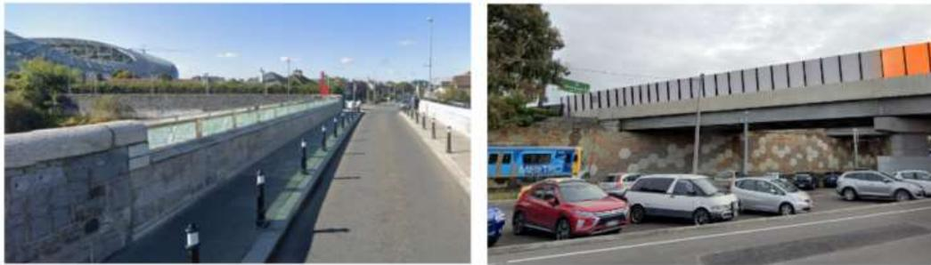
**Figure 4-6: Transparent or opaque parapet extensions (Glass – Dodder Bridge, Ringsend and Polycarbonate or Acrylic – Eastlink, Australia). Note that Section 4.3 of this report discusses relevant materials and recommends against the use of glass.**
