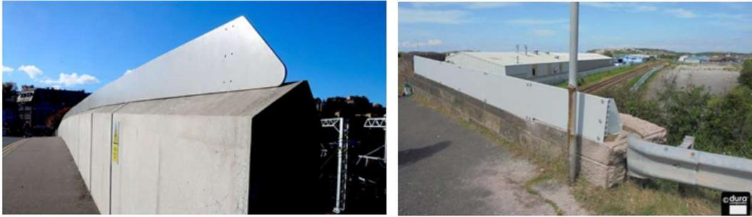
**Figure 4-5: Non-transparent parapet extensions (Steel – Bury’s Bridge, UK and GFRP example (source [www.duracomposites.com](http://www.duracomposites.com)))**
